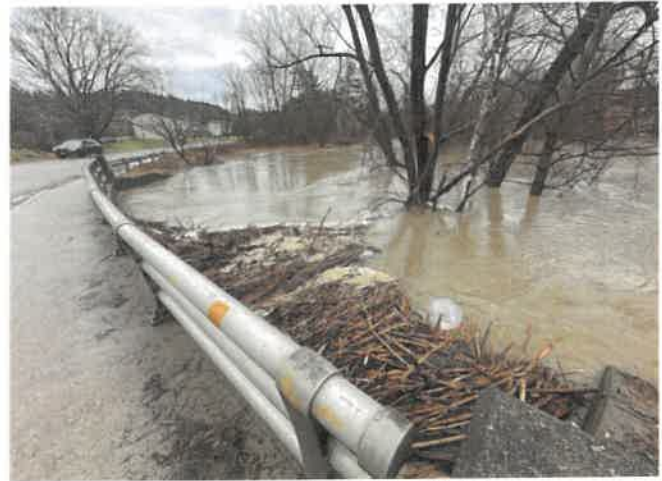
Armory Drive bridge near Union Street-photo by Gordon Miller
