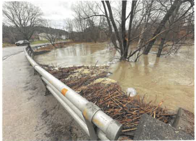
Armory Drive bridge near Union Street-photo by Gordon Miller
