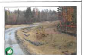
Filter Fabric and Stone Inlet Protection
