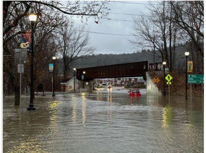
December of 2023 North Main Street. -Photo by Lisa Scagliotti from Waterbury Roundabout
