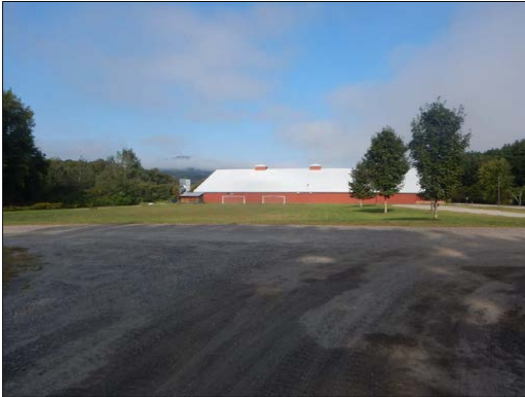
Photo 8. Ice Center property, note ice center building in the background and gravel parking area. View to the northwest.
