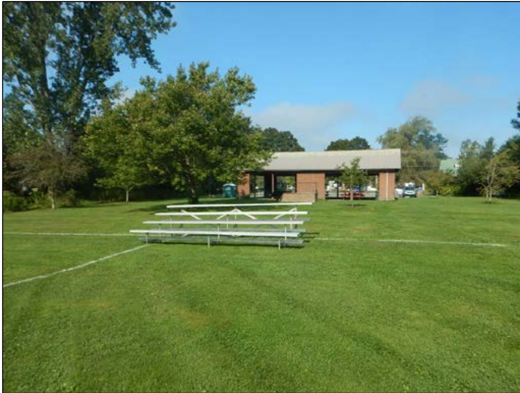
Photo 1. Hope Davey property, note highly landscaped playing field with pavilion. View to the northwest.
