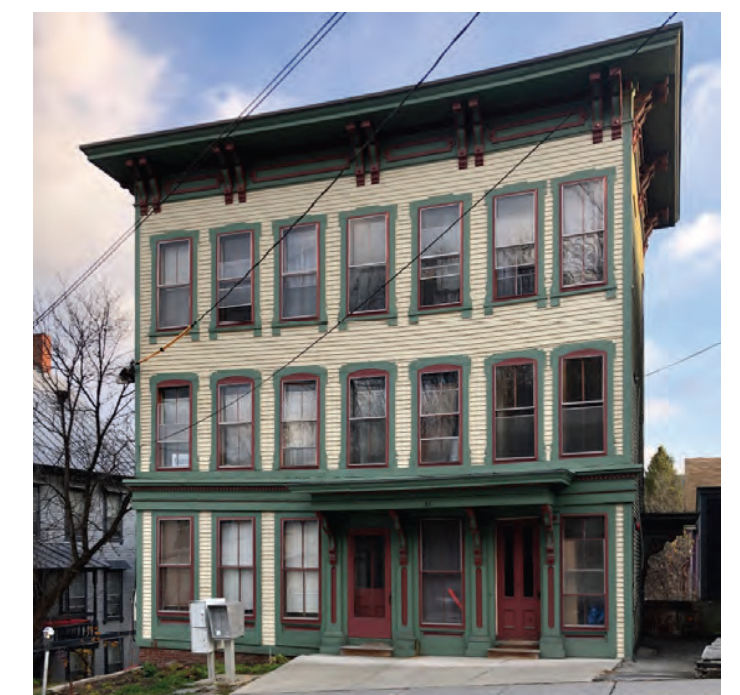
MULTI-FAMILY BUILDING MONTPELIER, VT
